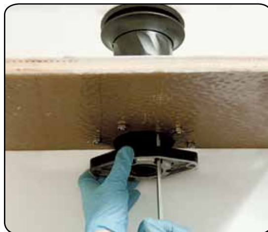
2. Tighten six M6 precote coated screws (8 Nm/ 71 in-lb)
